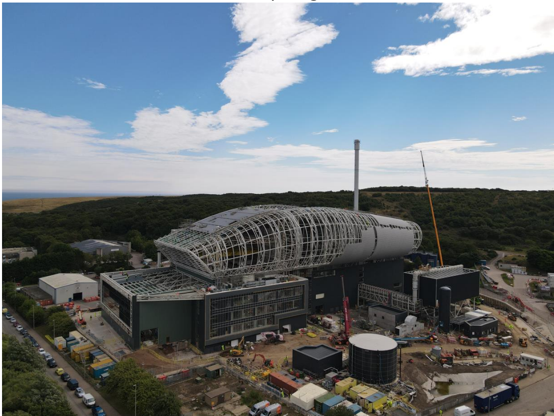
View from Northwest of the Facility: August 2022
